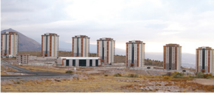
Gülkent Complex / KAYSERİ 15 Elevators, Rated Load: 630 / 800 kg
