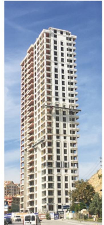
Selçuklu Towers / ANKARA 9 Elevators, 30 Stops, Speed: 2,50 m/s
