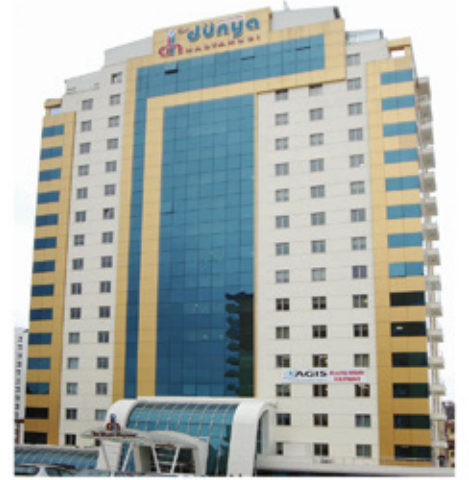
Dünyam Hospital / KAYSERİ 8 Elevators, Rated Load: 2000 kg
