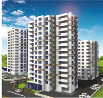
Ersu Construction Erkilet / KAYSERİ 8 Elevators, Rated Load: 800 kg
