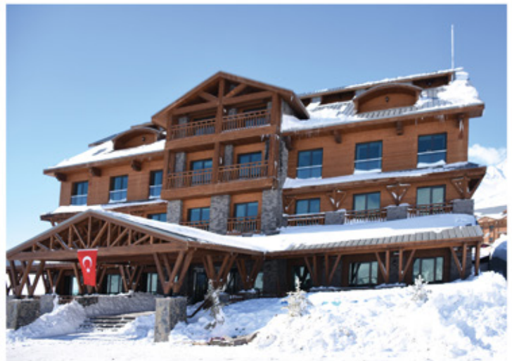
Magna Hotel / KAYSERİ 2 Elevators, Rated Load: 800 kg
