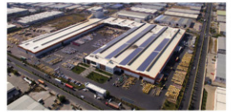
Haşcelik / KAYSERİ 3 Elevators, Rated Load: 800 / 3000 kg
