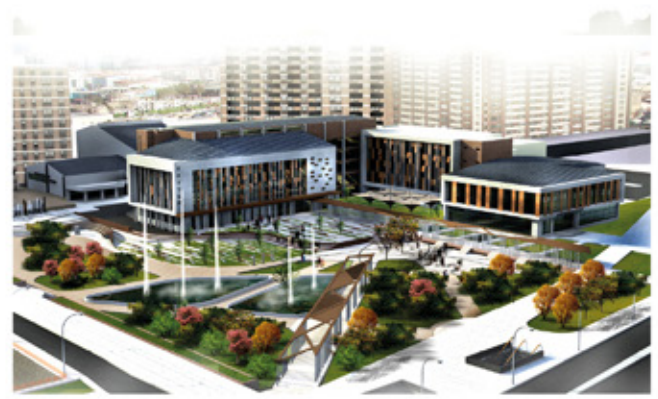
Kayseri Metropolitan Municipality / KAYSERİ Rated Load: 630 kg
