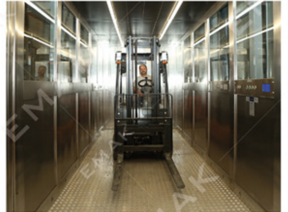
Çevik Warehouse - Showroom / ANKARA EMMAK Hydraulic Cargo Elevator Rated Load: 4 Tons
