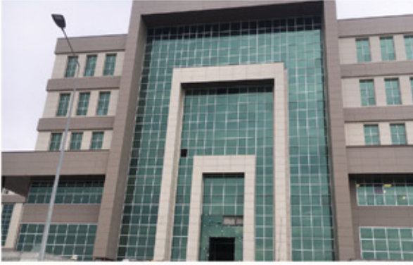
Courthouse / TEKİRDAĞ 15 Elevators, Rated Load: 800 kg
