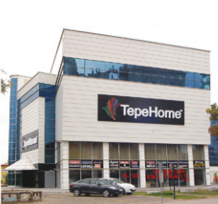
Tepe Home / KAYSERİ 3 Elevators, Rated Load: 1000 / 1600 kg
