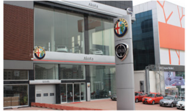
Akota Showroom / ANKARA 2 Elevators, Rated Load: 480 / 600 kg
