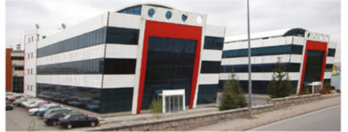
Deha Advertising / KAYSERİ 2 Elevators, Rated Load: 3000 kg
