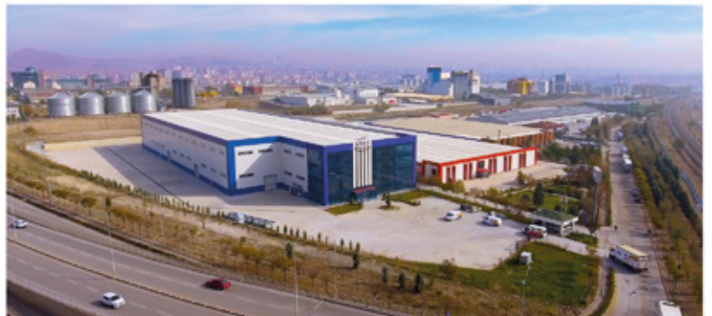
Seğmen Jam / ANKARA 5 Elevators, Rated Load: 450 / 3000 kg
